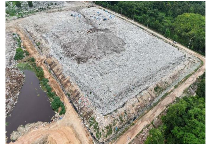
Waste pit no. 2
